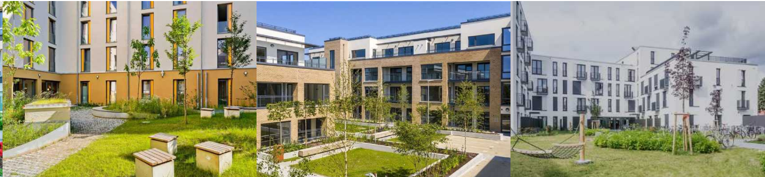
▲ Communal Area/Play Area - East of Apartment Block
